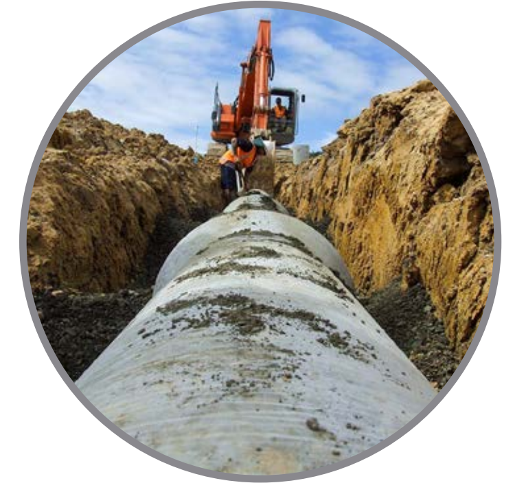
Pipe network upgrades
