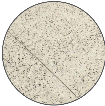
Main Pedestrian Circulation Exposed aggregate concrete
