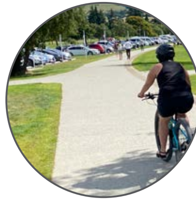
Shared Pathway Exposed aggregate concrete
